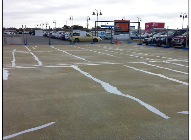
Crack repair to existing substrate
