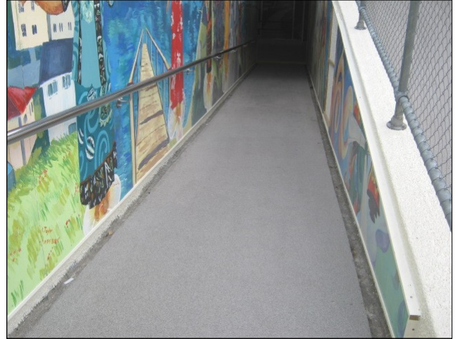
Entrance ramp completed with Duracon BC
