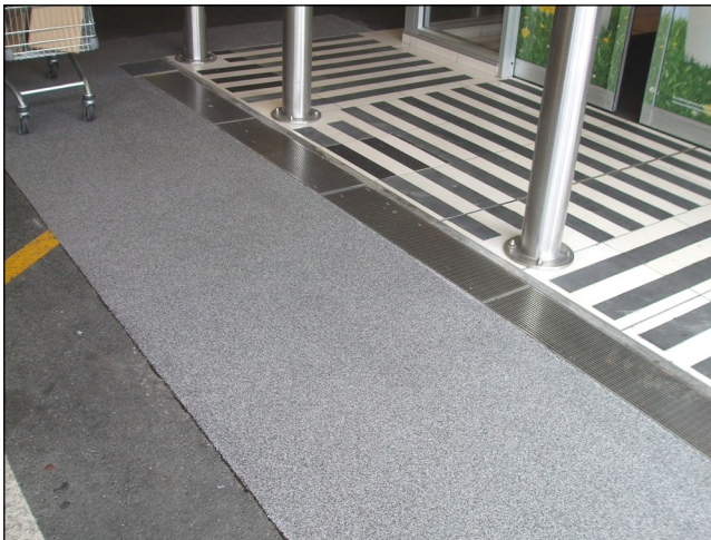
Completed Duracon BC Flooring System
