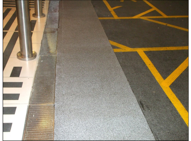
Duracon BC Flooring System applied to existing entrance
