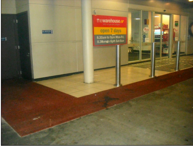
Entrance before refurbishment
