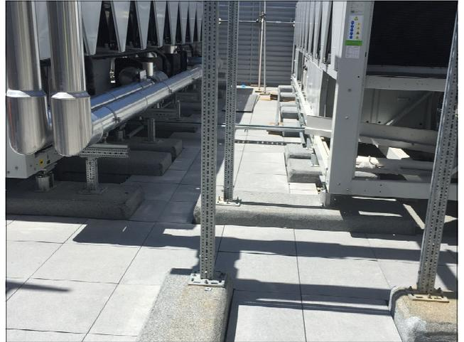
Completed DuO capsheet with pavers on plant deck
