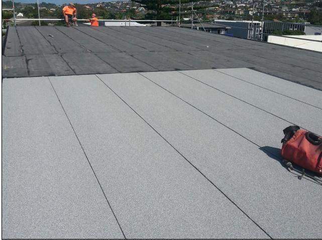
Application of DuO capsheet over basesheet and PIR thermal insulation board
