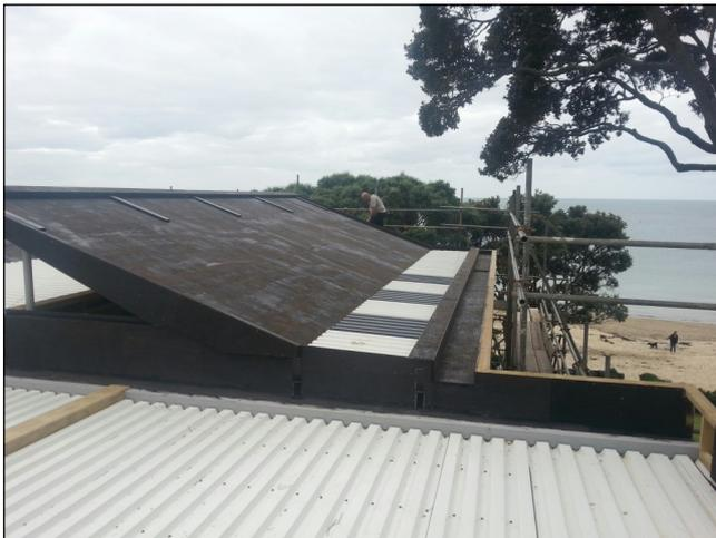
Substrate prepared for warm roof application
