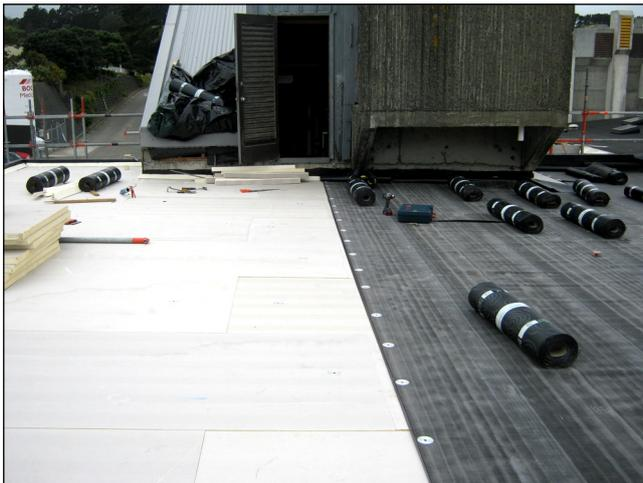
De Boer DuO basesheet mechanically fastened over Kingspan PIR Thermal Insulation board
