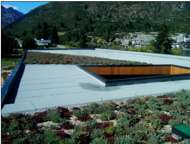
Finished project—mixed use roof concept
