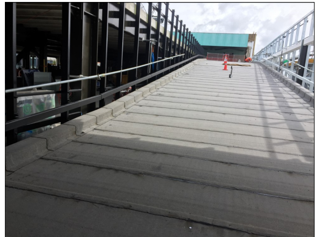
DuO 5mm Bridge & Tunnel membrane application to ramp
