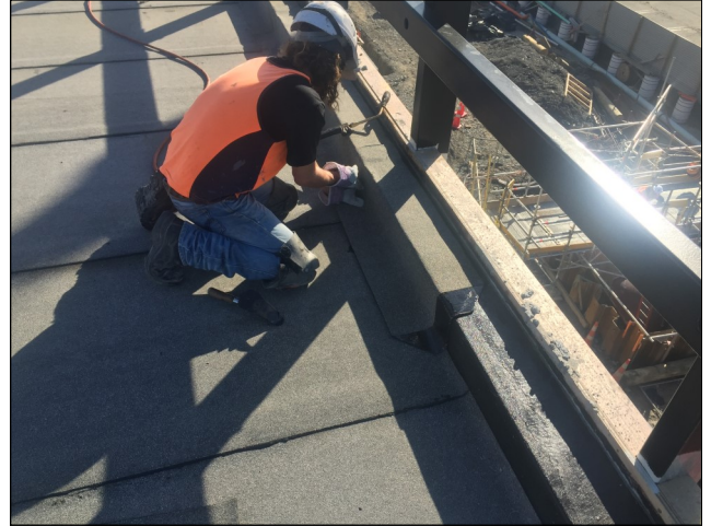
DuO 5mm Bridge & Tunnel membrane application
