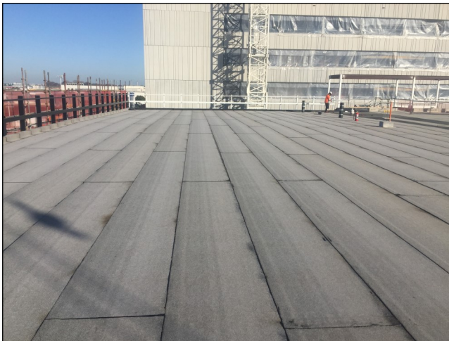
DuO 5mm Bridge & Tunnel membrane application to carpark
