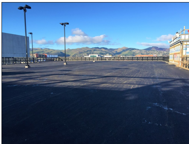
Asphalt installed on top of 5mm Bridge & Tunnel membrane
