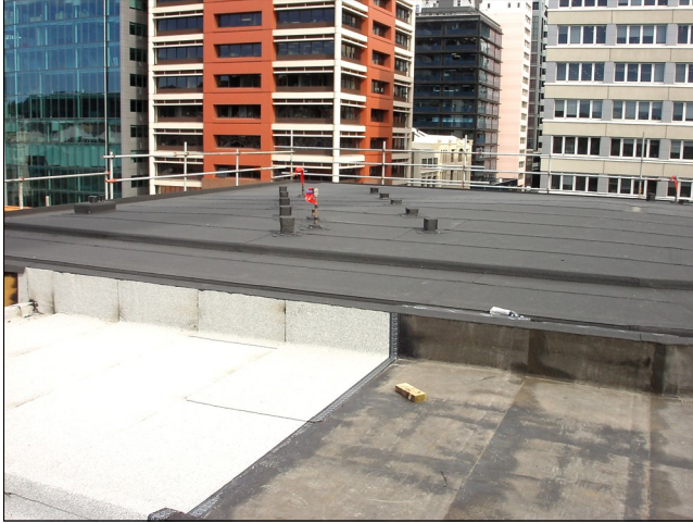
Basesheet membrane application
