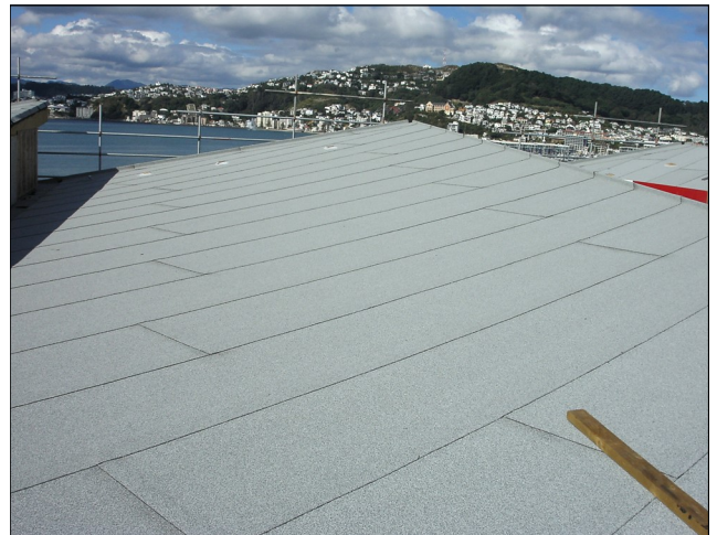
Finished De Boer DuO capsheet membrane
