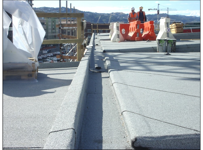
Gutter detail with De Boer DuO capsheet membrane
