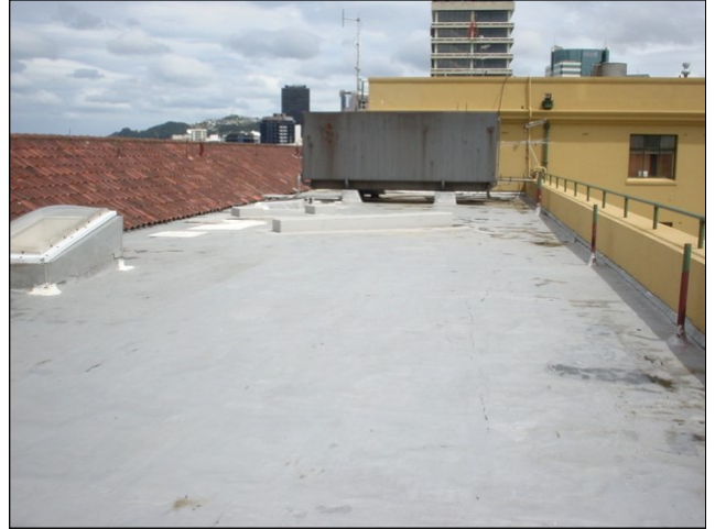
Existing roof before renovation
