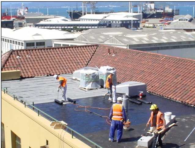
Preparation of area, primer and basesheet application
