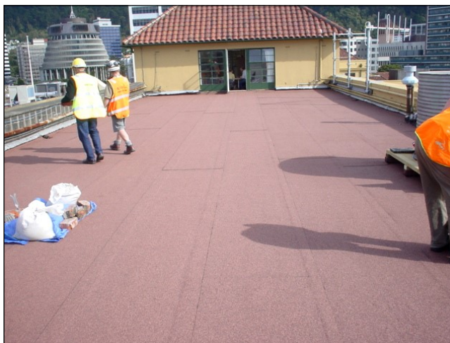
Completed roof refurbishment
