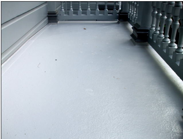
Finished Chevaline DEX Membrane
