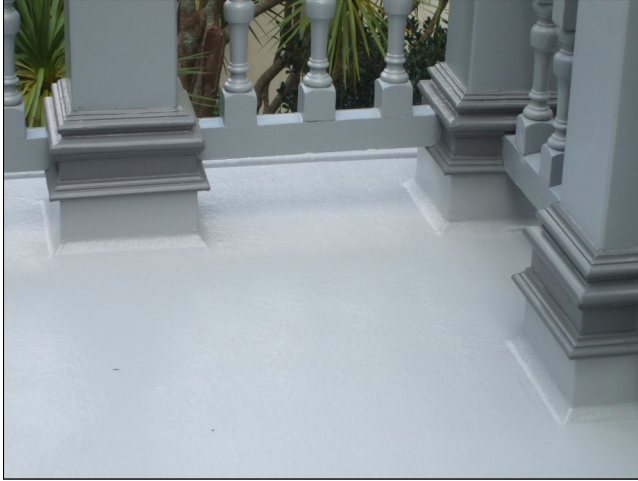
Finished Chevaline DEX Membrane detailing around upstand
