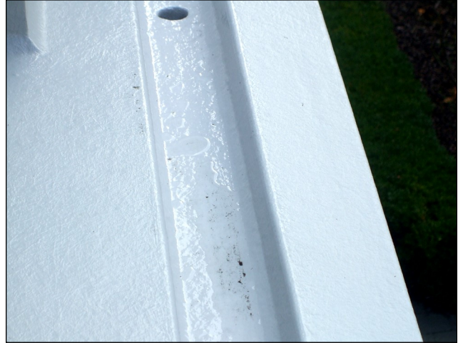
Finished gutter detail with Traxx 2000 wearcoat
