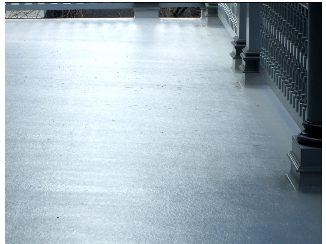
Finished Chevaline DEX Membrane
