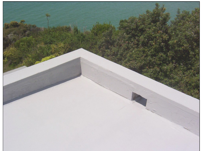
Detailing to parapet and scupper
