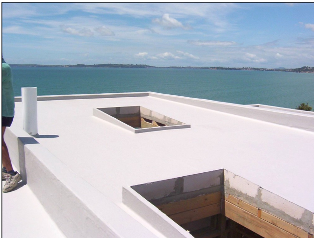
Dexx and fibreglass detailing around skylights
