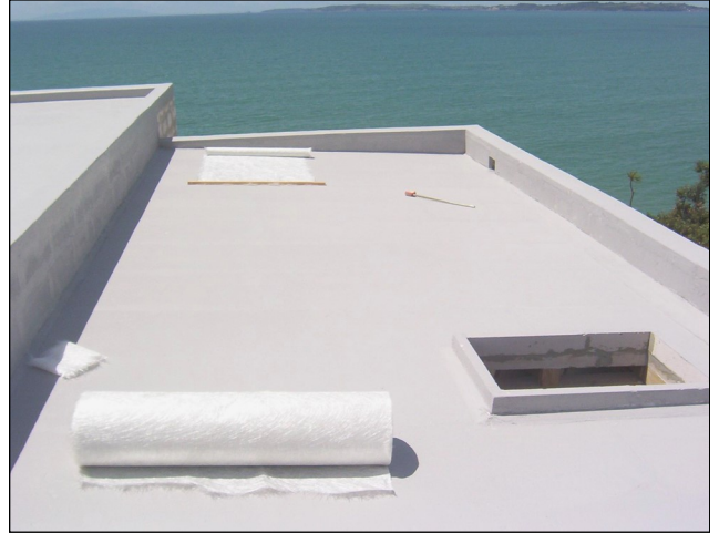
Fibreglass encapsulation into wet Dexx bodycoat
