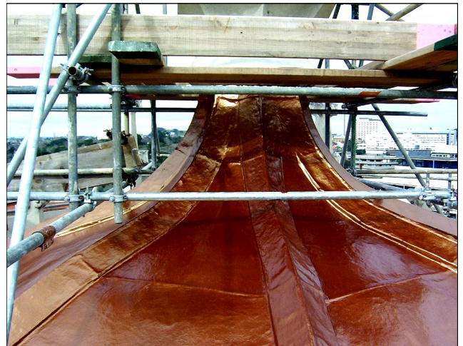
Chevaline Chemglaze protective clear finish applied
