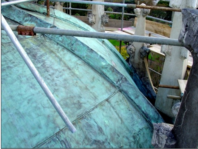
Original weathered copper roof
