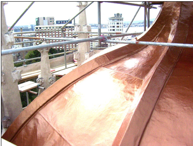
Copper Dexx Bodycoats with Fibreglass reinforcement
