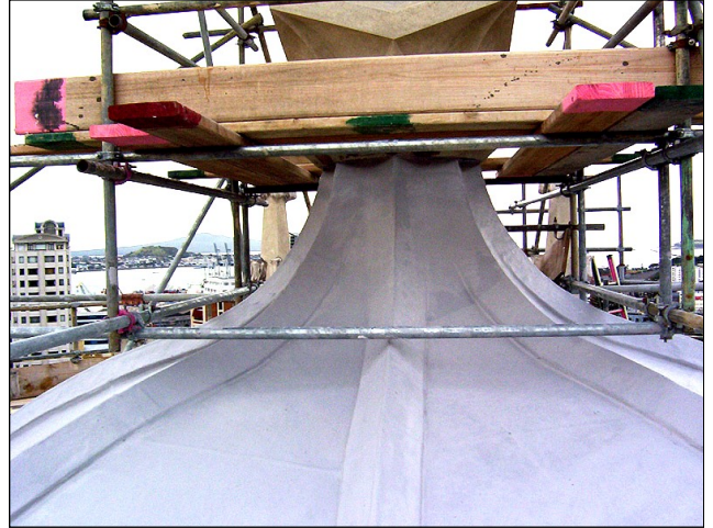
Chevaline Dexx base coat applied over copper
