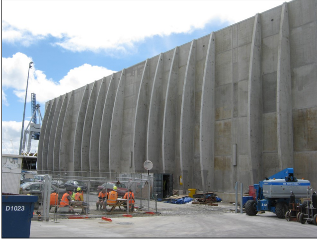
Substrate prior to cleaning and preparation
