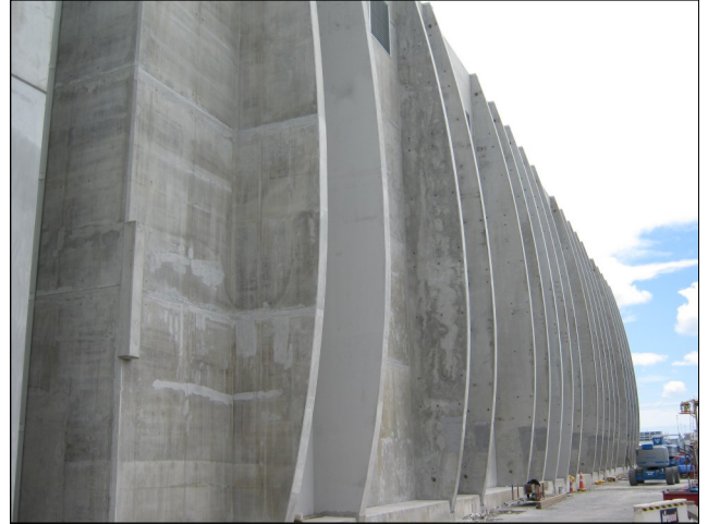
Trial fin completed
