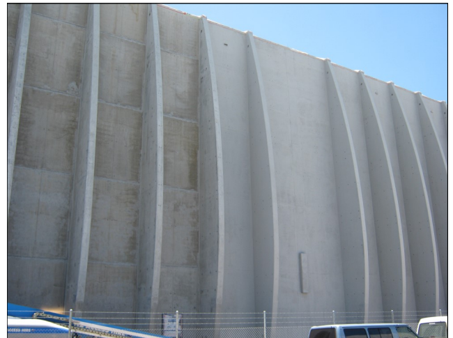
Close up comparing uncoated and coated work
