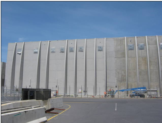
Application of Concretal Lasur by airless spray
