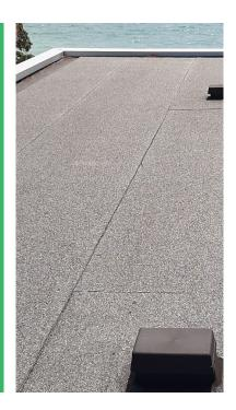
The Polibit Mineral Membrane System consists of a Polibit Mineral cap sheet torched to a 3mm self adhesive (SBS) base sheet, to form a two layer waterproofing membrane system suitable for flat roof waterproofing.
