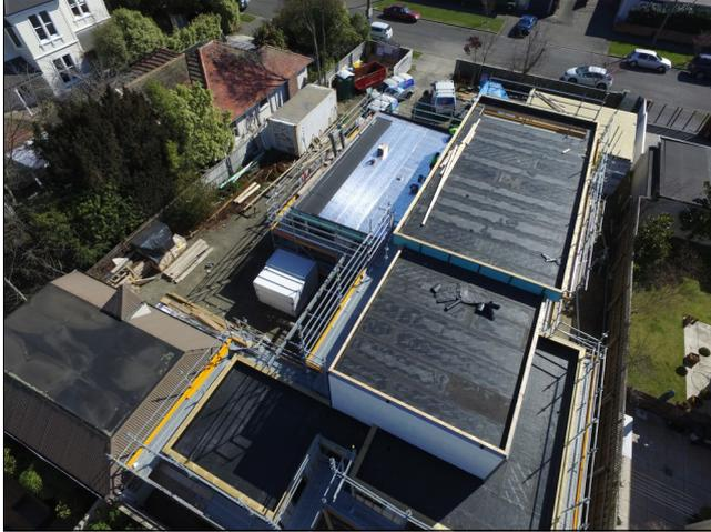
Vapour barrier installed over plywood substrate
