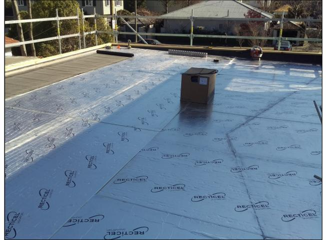
Recticel PIR insulation board installed over vapour barrier
