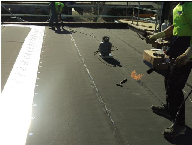
Basesheet mechanically fastened to PIR board
