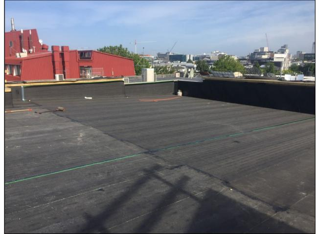
DeboTack Aero self adhesive basesheet applied over PIR thermal insulation board
