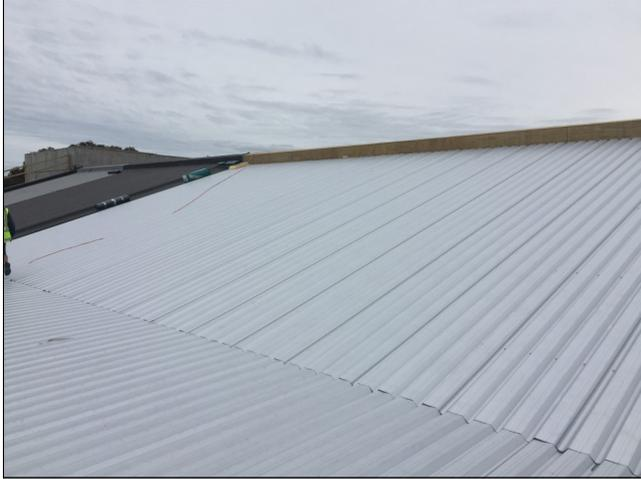
Metal substrate ready for warm roof installation
