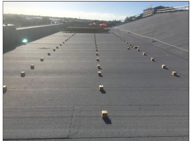
Finished DuO capsheet application with nib installation for Solar Panels
