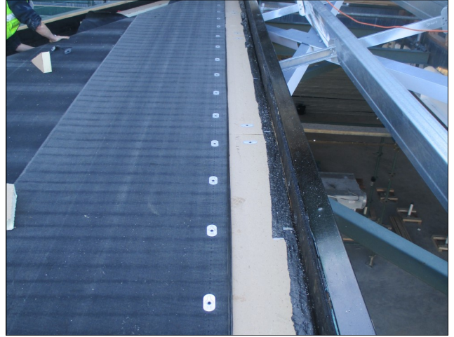
De Boer basesheet mechanically fastened over PIR thermal insulation board
