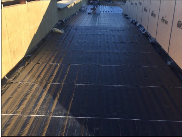
Vapour barrier applied to metal tray substrate
