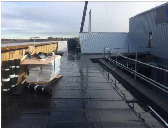
Basesheet ready for De Boer DuO capsheet application
