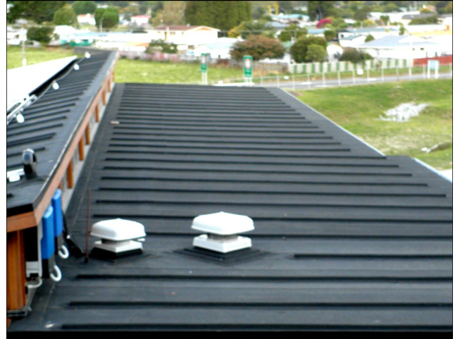
Completed DuO membrane roof
