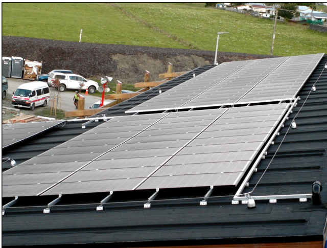
Completed DuO membrane roof with solar panels
