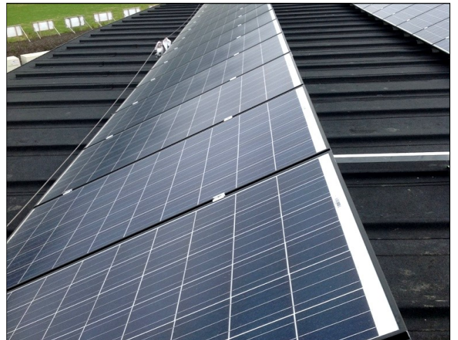
Completed DuO membrane roof with solar panels
