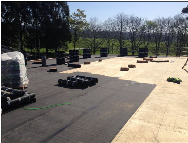
Plywood substrate with vapour barrier application
