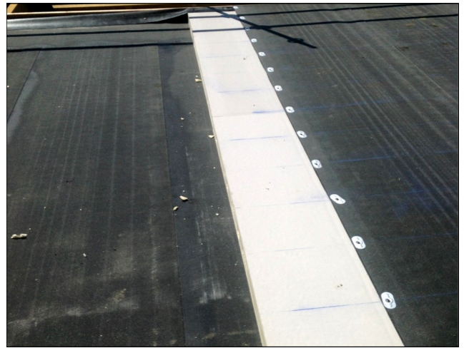
De Boer Basesheet mechanically fastened over PIR thermal insulation board and vapour barrier
