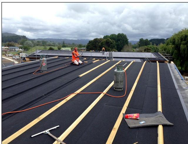
De Boer DuO capsheet and batten installation
