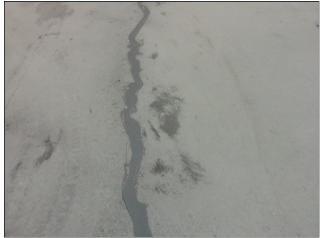
Crack repair
