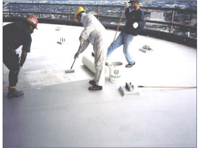
Installing fiberglass reinforcement into Dexx system
